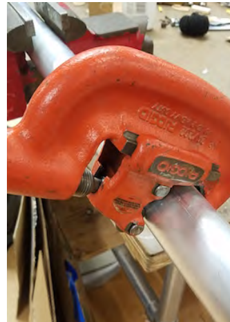
Cutting the steel rods to size.
